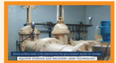
The well will be equipped with Aquifer Storage and Recovery (ASR) technology to allow surface water to be injected into the groundwater aquifer for storage and recovered for future use. This allows us to practice conjunctive use - using more groundwater in drier years to save surface water, and in wet years, using more surface water to allow the groundwater aquifer to recharge over time.
